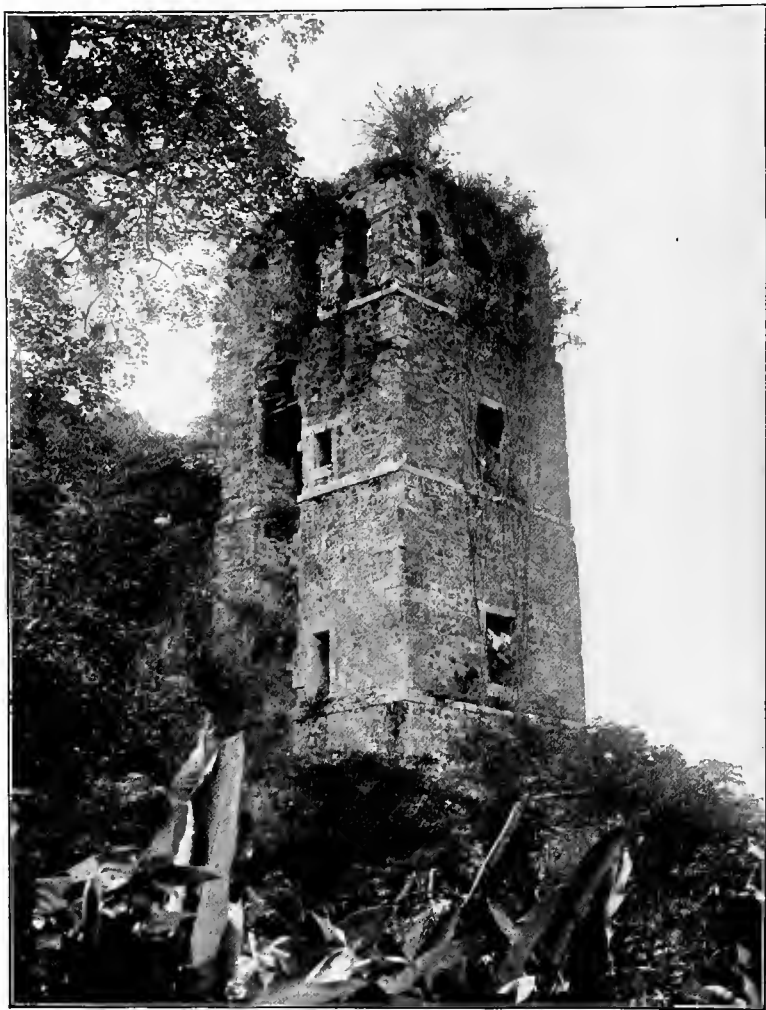
MASSIVE TOWER OF SAINT AUGUSTIN.
