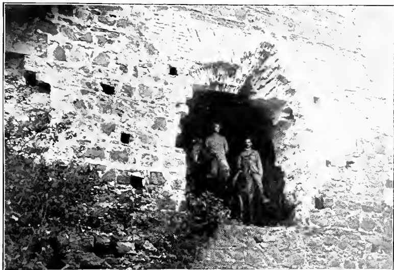
WALL OF TOWER OF ST. AUGUSTIN.—NOTE THICKNESS OF MASONRY.
